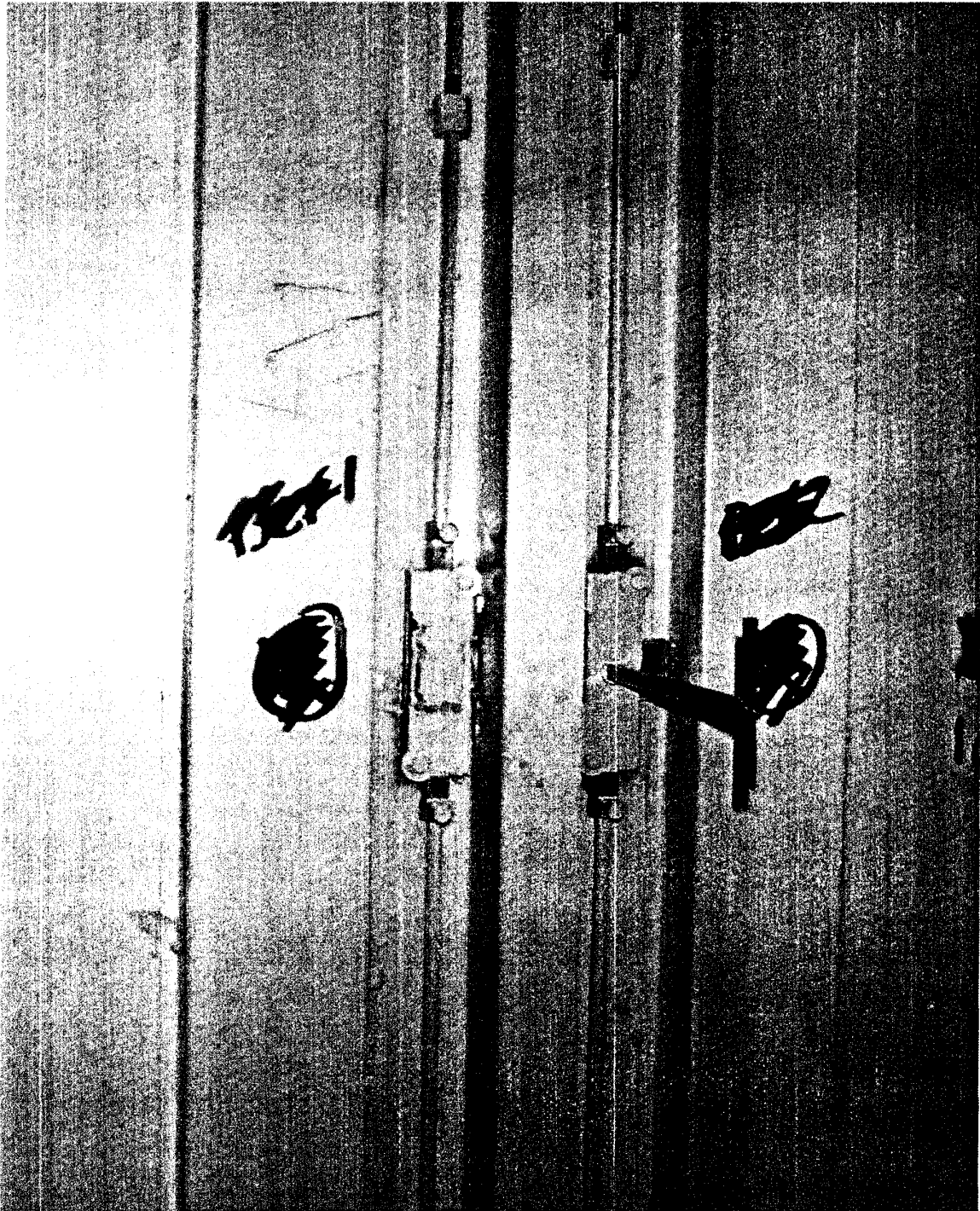
Photograph 3 Showing the two point and three point locking mechanisms used on the access panel door.
