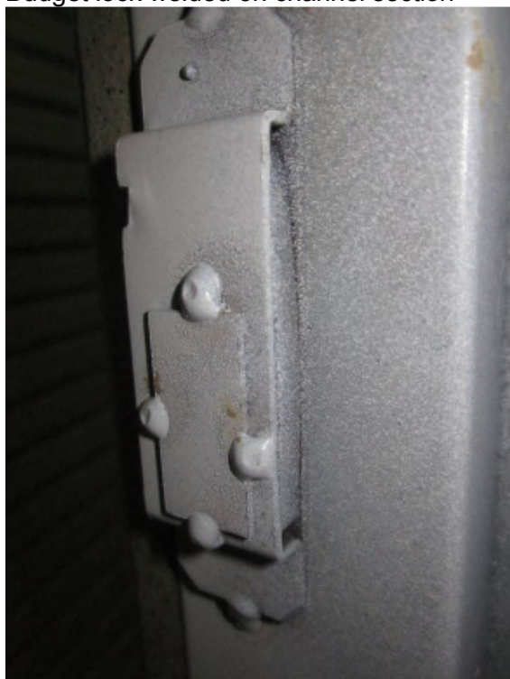
Budget lock welded on channel section
