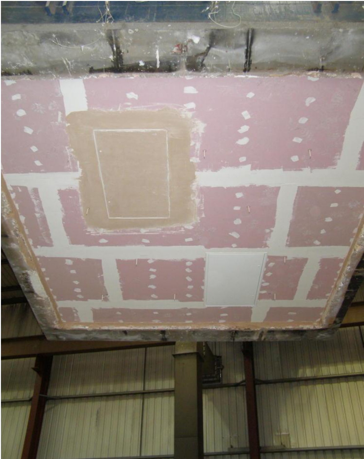
Exposed face of ceiling before test.
