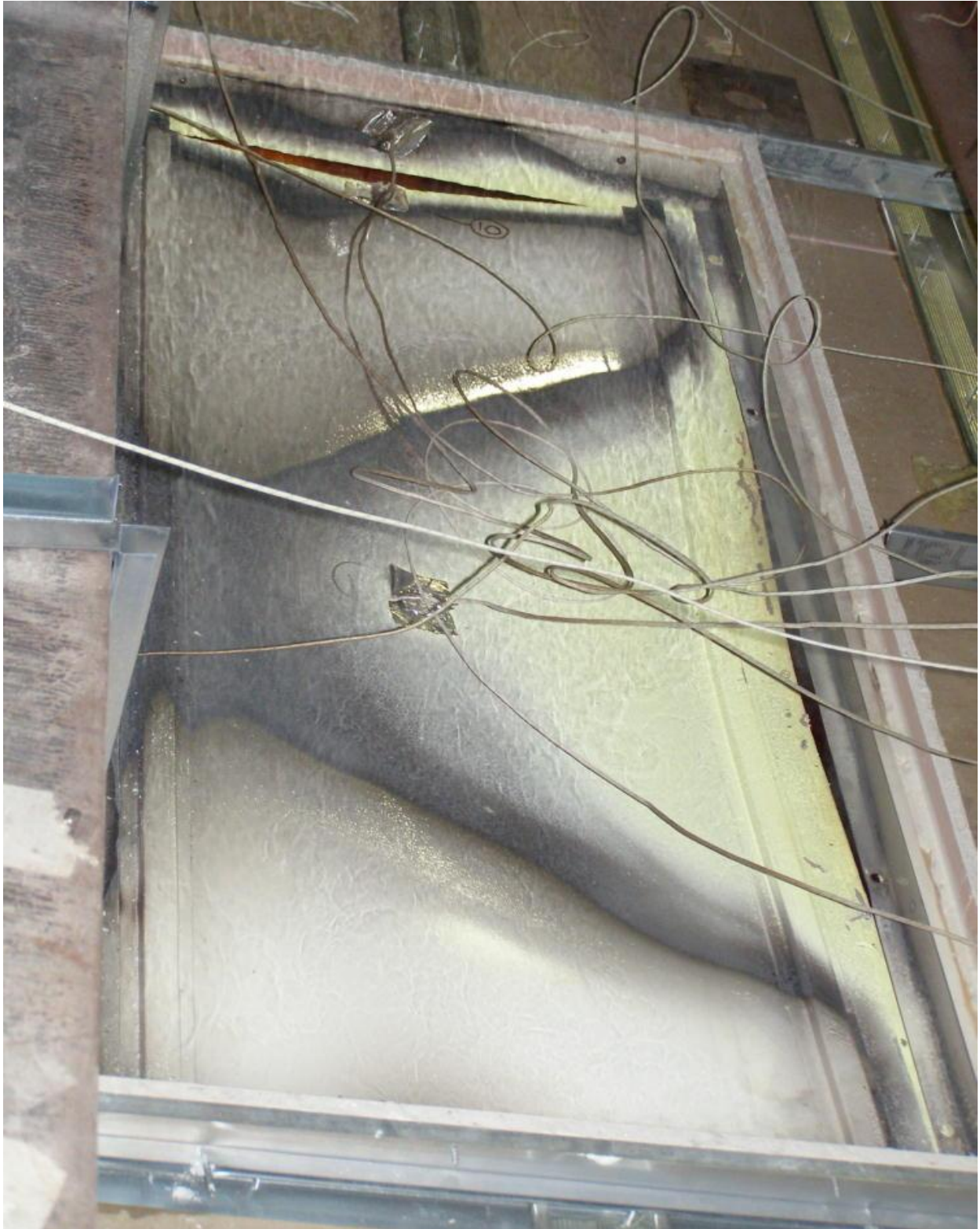
Unexposed face of ceiling showing PFBF access panel after 30 minutes.
