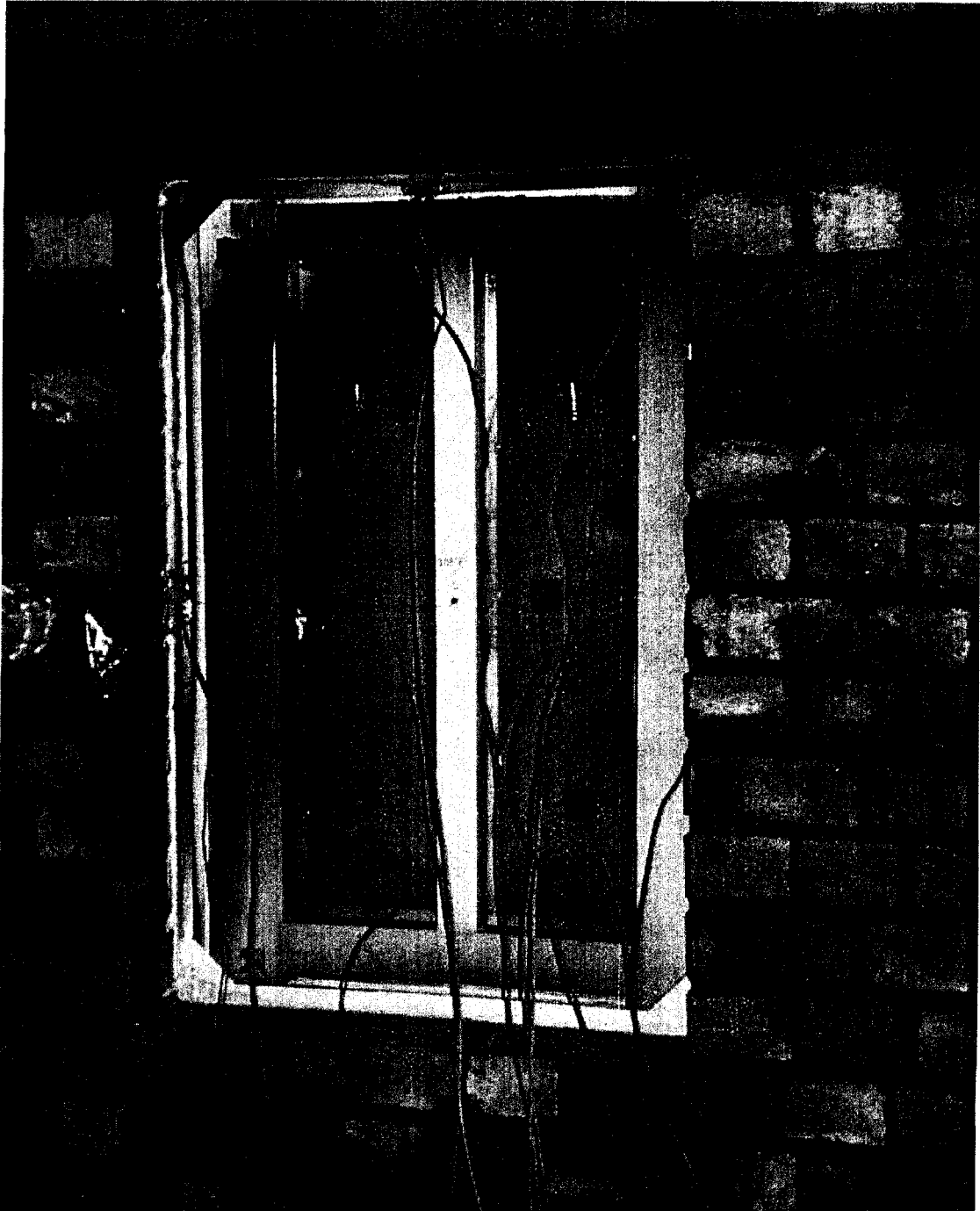
Photo 3 Unexposed face of specimen after 60 minutes.
