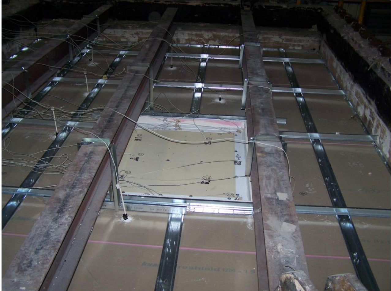
Unexposed face of ceiling before test.
