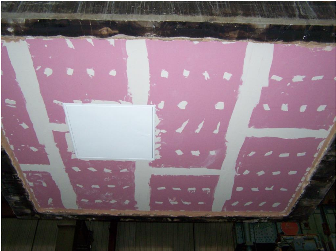
Exposed face of ceiling before test.
