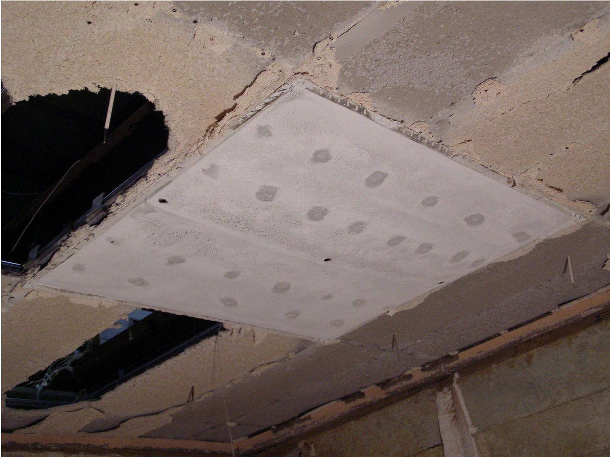
Photo 5 Exposed face of access panel after test.
