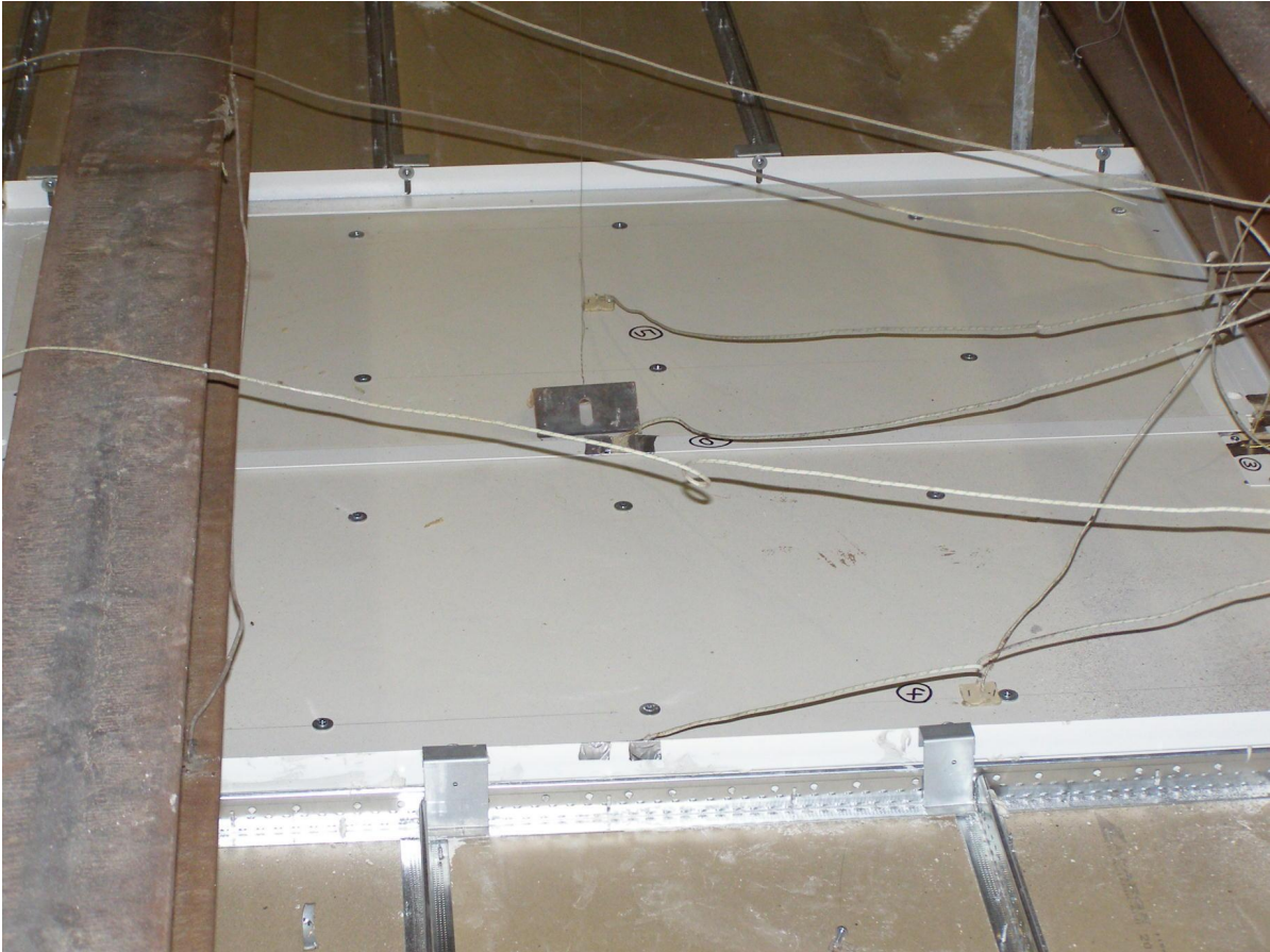
Photo 3 Unexposed face of access panel before test.
