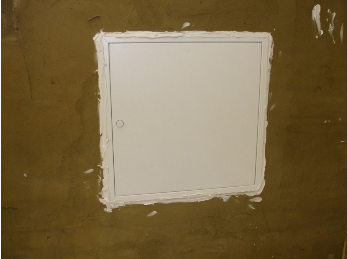
Photograph 1 – Test 2 – View from receive room
